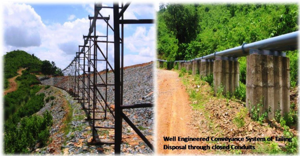
Conveyance System for Tailings
